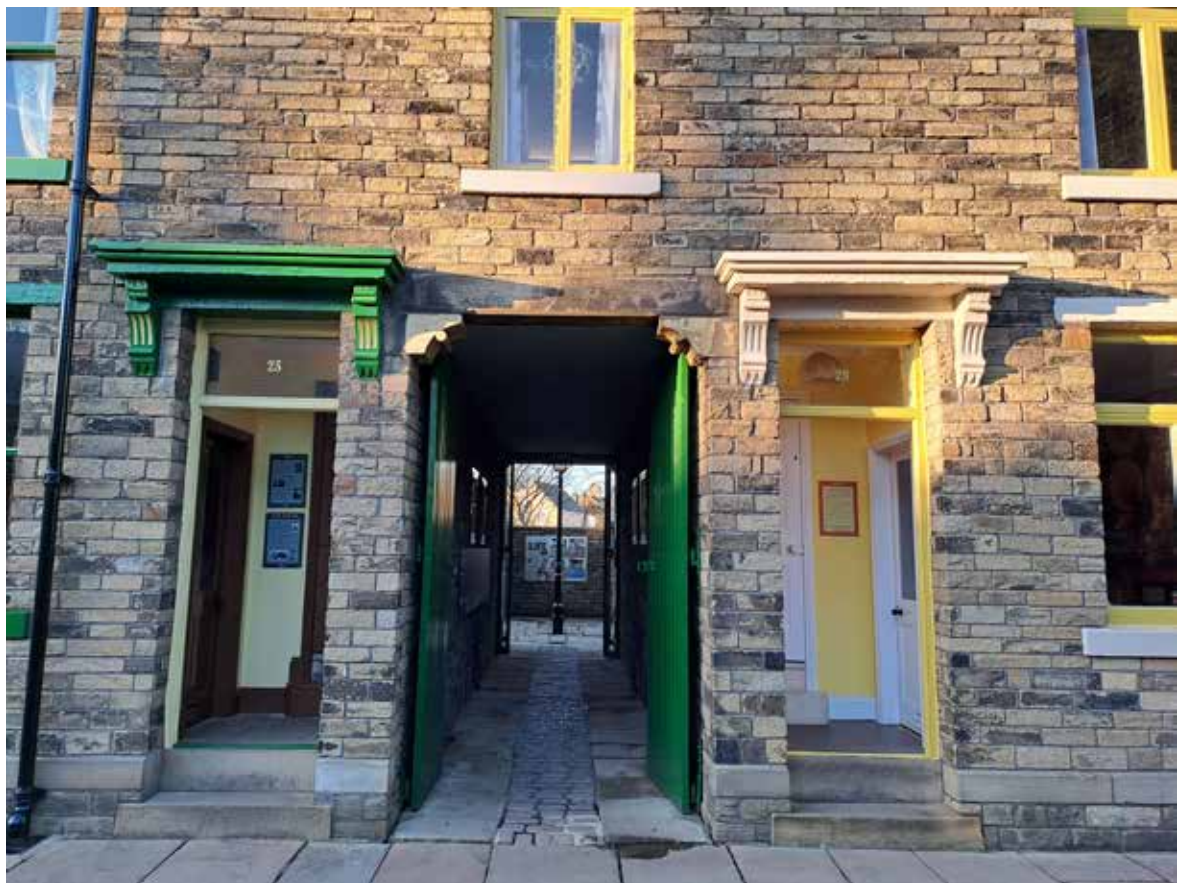
The front entrance of the Back-to-Back Terraced Houses.
